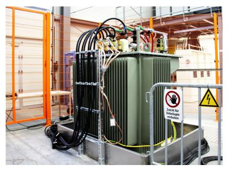
Prototype of a controllable MV/LV transformer made by J. Schneider Elektrotechnik GmbH. Tests in SysTec for the Project "Aktives, intelligentes Niederspannungsnetz"
