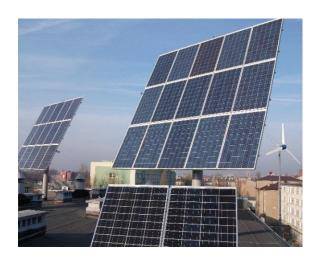
Sun tracking PV system 9 kWp
