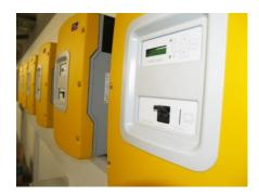
The two 25 kW FLA battery bank are connected to two three-phase groups of grid forming inverters – SMA Sunny Island inverters, enabling:
