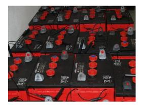
25 kWh capacity Flooded Lead-Acid (FLA)
